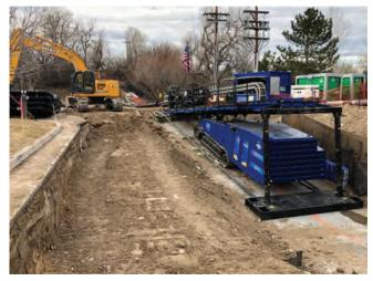
was completed using horizontal directional drill (HDD) equipment with the capacity to pull the nearly 2,346 m (7,700 linear ft) of heavy-wall HDPE pipe and associated drill stem through the tunnel. The pipe consisted of 122-cm (48-in.) diameter SDR 13.5 IPS HDPE (PE 4710) with a wall thickness of approximately 9 cm (3.6 in.) and a weight of 218 lbs/ft.
