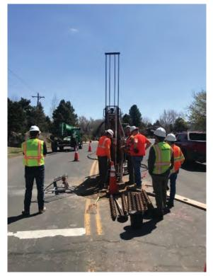
(3-in.) steel casing pipe along the entire length of the newly drilled grout injection points. Pressurized flow was achieved at the existing vent shafts by installing a sewer plug with a bypass hole. The grouting pressure was monitored at the ground surface utilizing a pressure gauge on the injection stack, and the allowable pressure was calculated for each injection point based upon the vertical depth (head) to the HDPE pipe.
