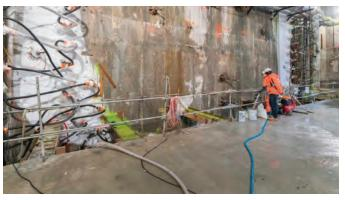
In order to reduce water inflows inside the excavation area, tube-a-manchette injections were performed between the frozen body and the RER base slab. Several drains had to be installed to lower the water table because permeability criteria were not reached in the grouted area. These drains were active from the beginning of the excavations to the end of concreting works.
